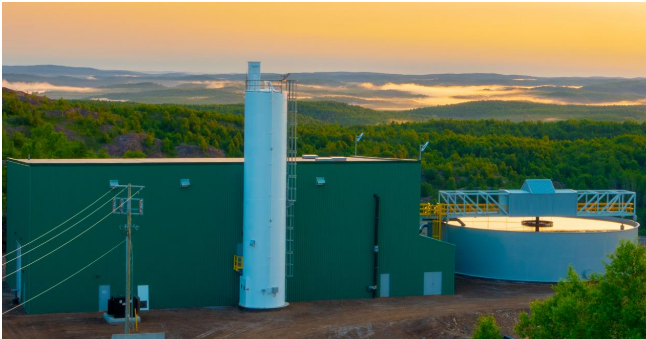
Photo 1. The MacLeod HDS Plant
